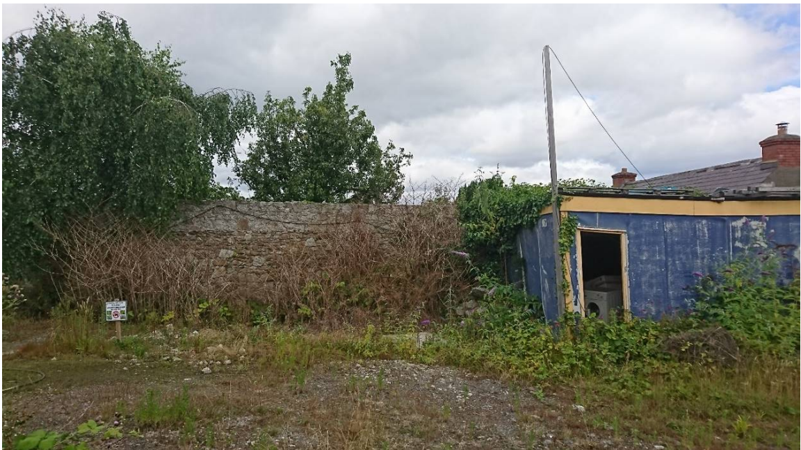
Plate 16.5 - Stone bonded wall to southeast of Grange Cottages, facing northwest
