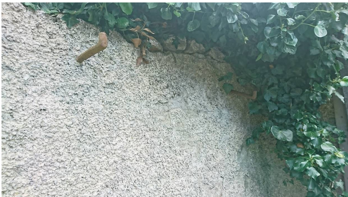
Plate 16.10 - Metal fixtures in wall, facing east
