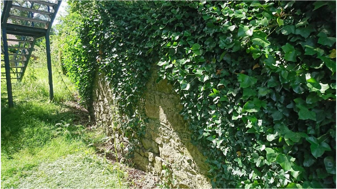
Plate 16.16 - Wall along southwest boundary in Section Two, facing south-southwest
