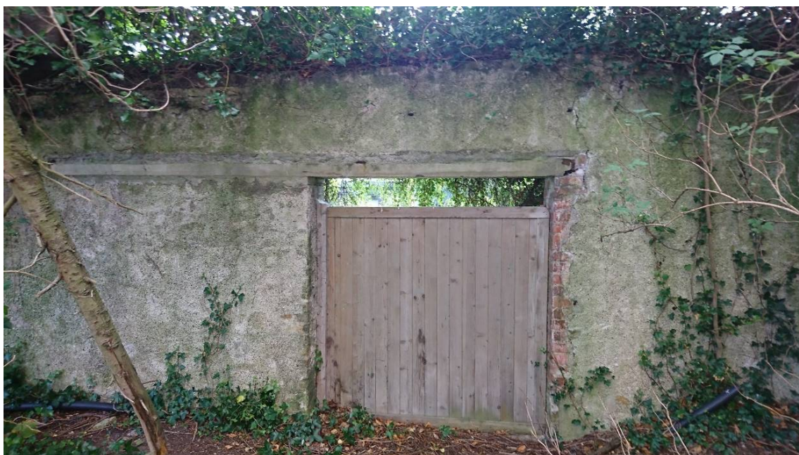
Plate 16.9 - Entrance in wall opposite the abandoned building complex, facing northeast
