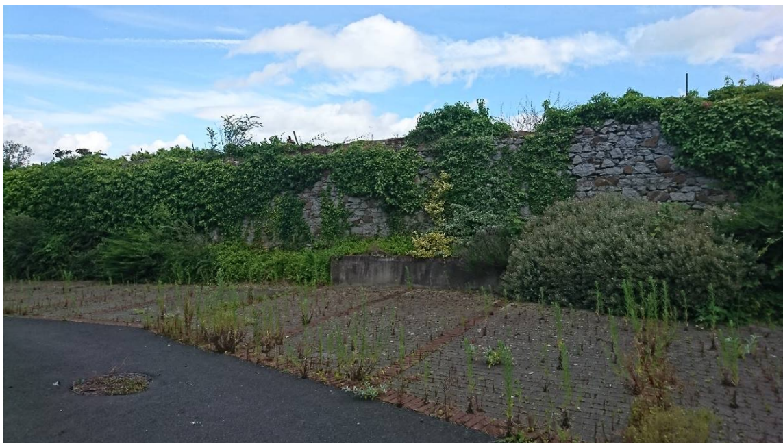
Plate 16.12 - Stone wall dividing Section One and Two, facing north-northeast
