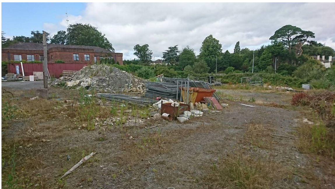
Plate 16.1 - Section One western portion, facing northwest
