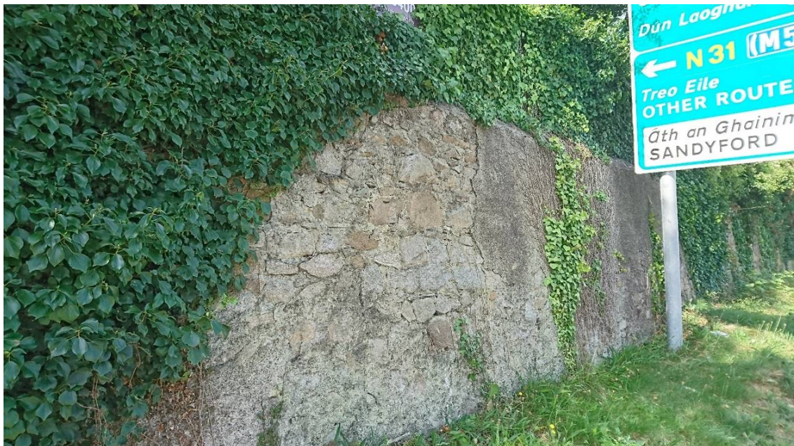
Plate 16.7 - Wall fronting onto the N11 from Section One, facing northwest
